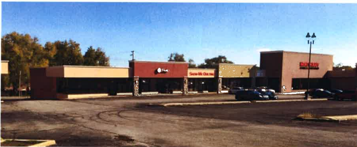
Figure 1 – View of South Building of Raytown Plaza Shopping Center
